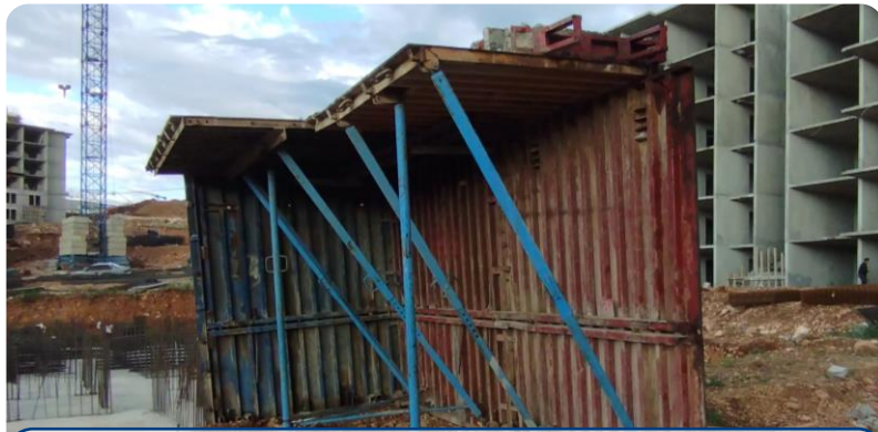
Modular, prefabricated tunnel-formworks tailored to particular project
