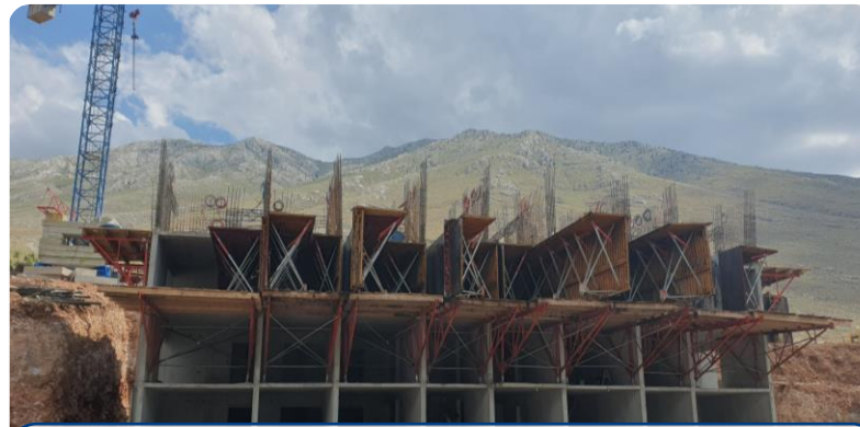
Monolithic casting of a single story in one pouring operation
