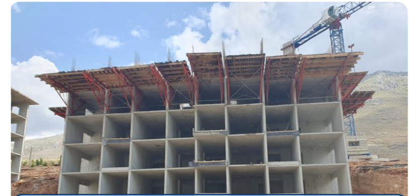
Easy stripping, high mobility and re-use of formworks
