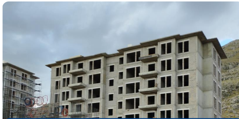
A particular architectural form constrained by the tunnel-formwork application
