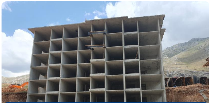
Lightly reinforced slender shear walls, squat coupling beams, and thin slabs
