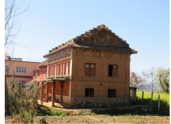
Brick with mud mortar (BrM)
