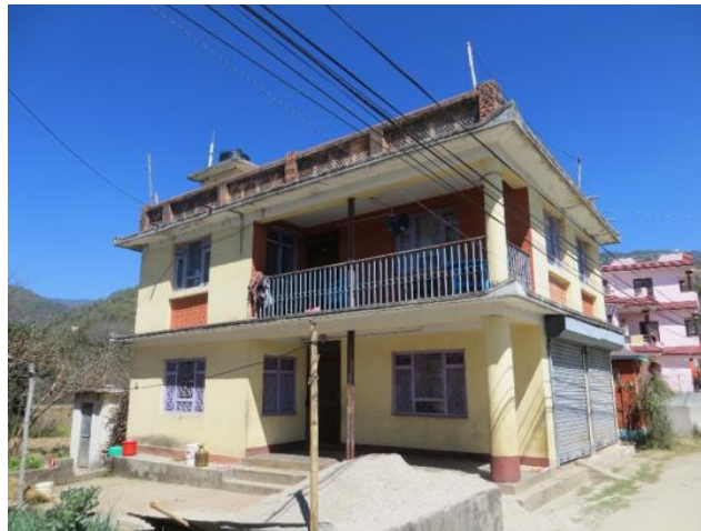
Brick in cement with rigid diaphragm (BrCri)
