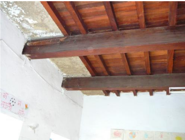
Brick in cement with flexible diaphragm (BrCfl)
