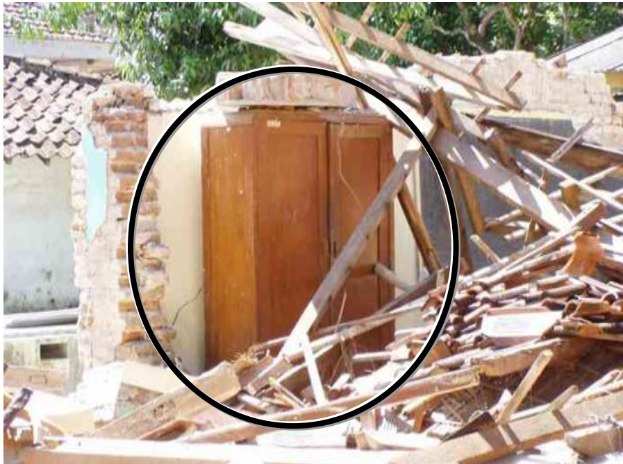
An elementary school damaged by the Central Java EQ 2007, Indonesia
