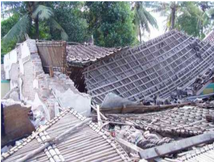
Unreinforced brick masonry in Indonesia
