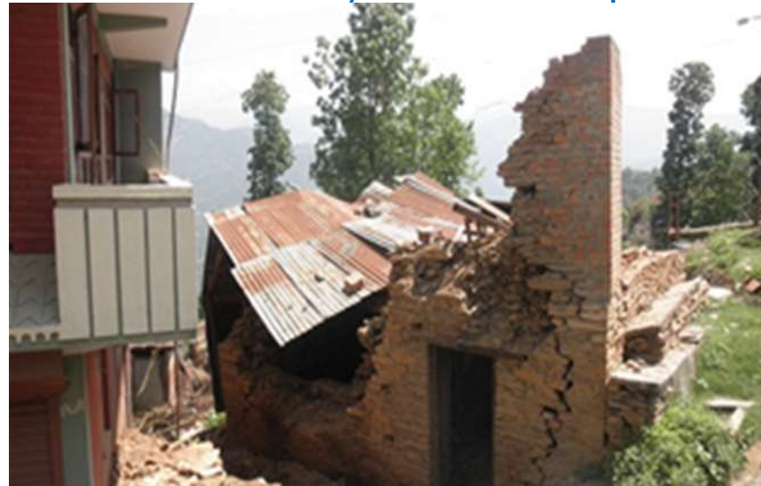
Stone masonry house in Nepal
