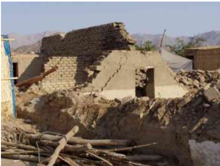
Adobe houses in Peru
