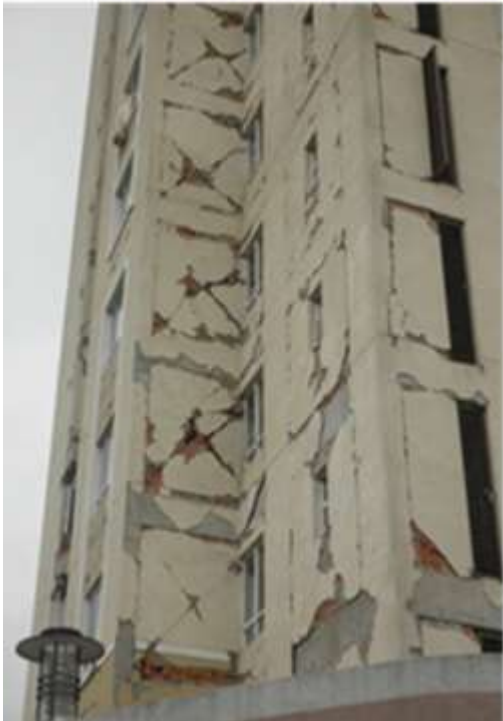
Most of high rise apartment houses in Kathmandu got heavy damage in non-structural walls by Gorkha EQ 2015
