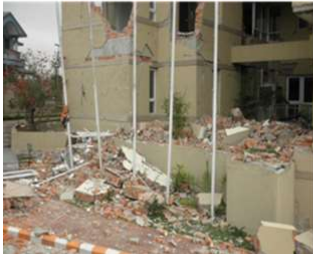
Most of high rise apartment houses in Kathmandu got heavy damage in non-structural walls by Gorkha EQ 2015
