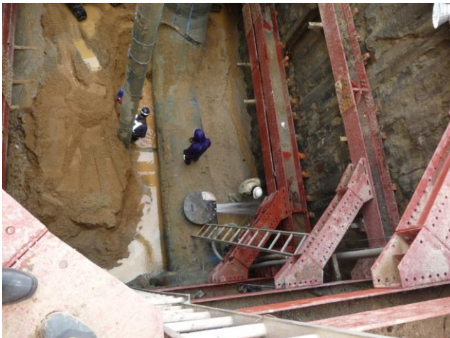
2016 Kumamoto EQ. Steel pipe ( \phi 1350 mm) deployed in 1982
