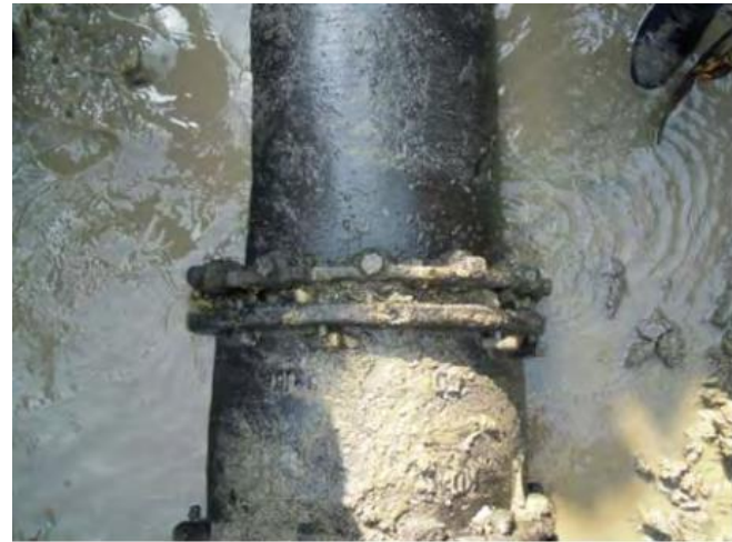
2011 Tohoku Japan EQ. Ductile cast iron pipe (K-type, \phi 500 mm) deployed in 1974
