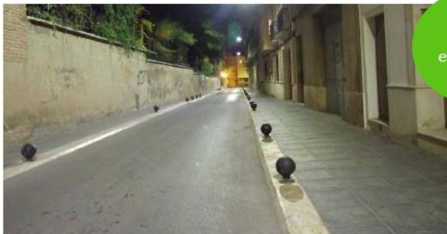
31W NW MSO H:6m, S:21m, Ancho 3m Ehmed 11lux, U_o = 0.6 Ra 70 IRC: 70; Tc 4000K
