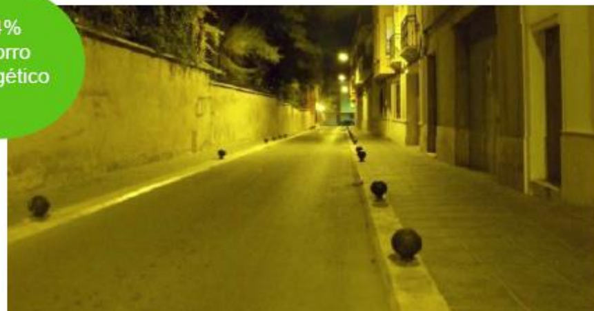
SON100W PC (120W medidos) H:6m, S:21m, Ancho 3m Ehmed 19lux, U_o = 0.3 Ra 20 IRC: 25; Tc 2100K
