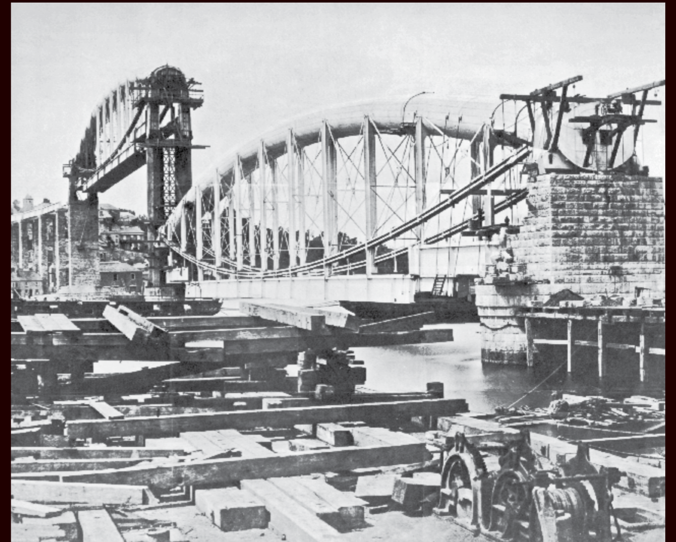
Royal Albert Bridge
