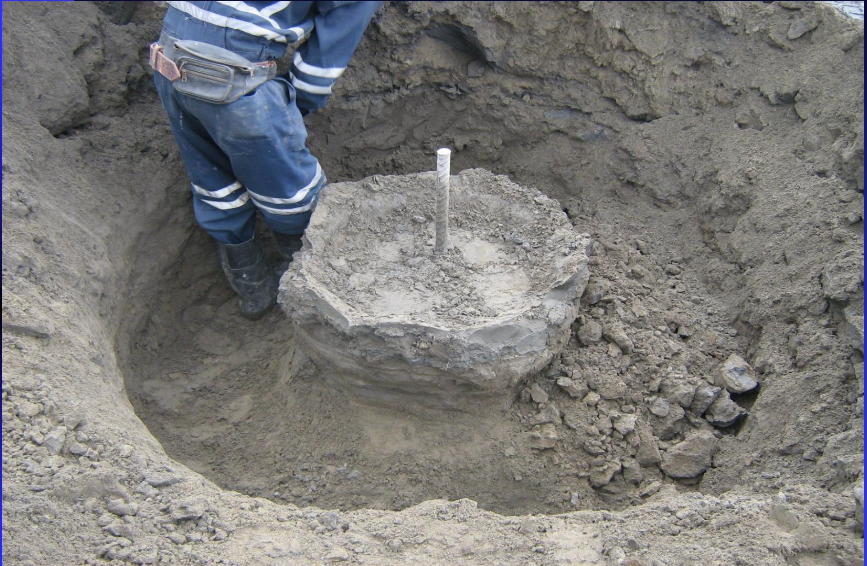
COLUMNA JET GROUTING INSTALADA
